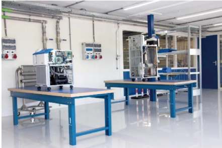
Chiller Repair Center
