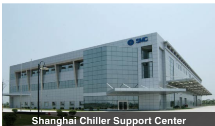
Shanghai Chiller Support Center
