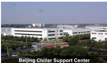
Beijing Chiller Support Center
