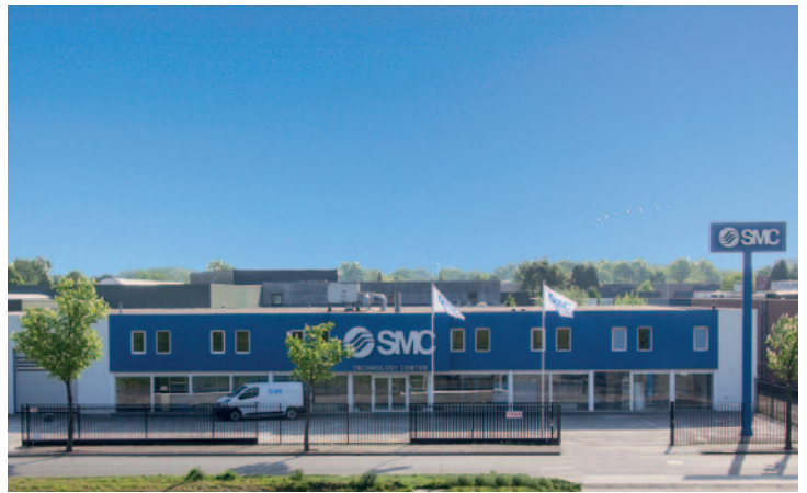
The SMC Technology Center in Eindhoven.
